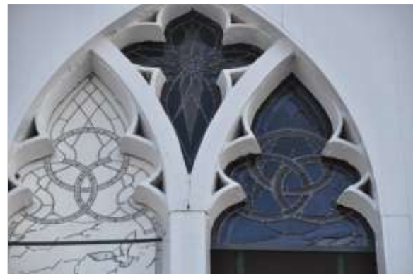
Boards depicting the window design were in place for 8 months during window production. Installation of the stained glass pieces began at the top.
